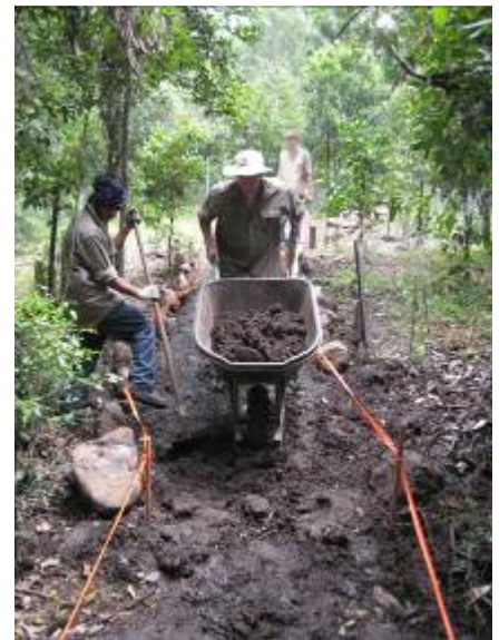
Nathan brings in another barrow load of fill while Johnny is on rake duty.
